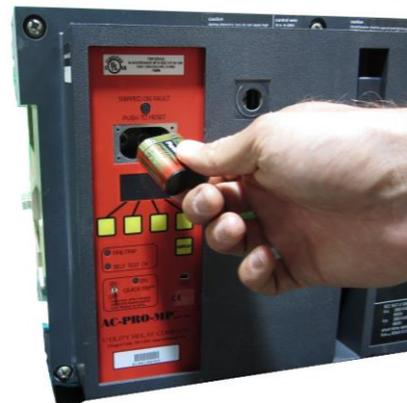
Remove the old battery and install a new CR-P2, 6 Volt Lithium battery. Replace the battery cover.
